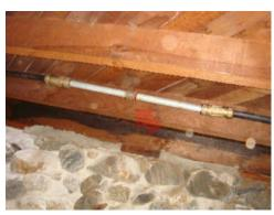
[CR] The kitchen dishwasher water is supplied with plastic tubing from the water heater hot supply line. A shutoff valve is not provided.
