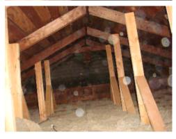
This area of the roof framing at the front right appears to have been where a masonry chimney was removed.
