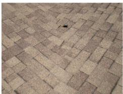
[CR] The front lower roof is lacking proper valley flashing. Improper installation of the shingles at this location.
