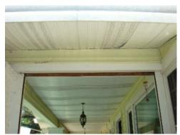
[CR] The front pot shelf slopes towards the wall improperly, and the siding is separated.
