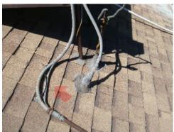
[FE] [CR] A low voltage wire is scorched and damaged at the unit cabinet wall. The wire is lacking a bushing for protection.
