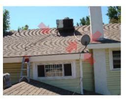
[CR] The A/C condensate drain line terminates improperly at the upper roof edge. Roof gutters should be installed to direct the condensate water to the driveway.
