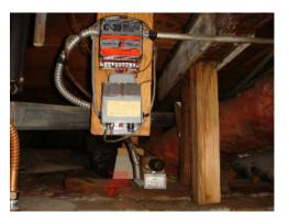
[SC] [FE] [CR] [RU] The original knob & tube wiring has been spliced into improperly with updated wiring, in the attic, basement and garage.
