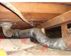
[CR] The abandoned registers should be sealed off, and the ducts sealed off in the craw space to prevent air transfer.
