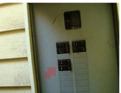
[CR] The added device is improperly wired to the main service conductors.
